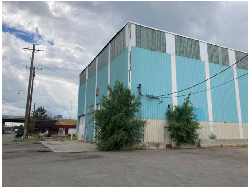
(existing site conditions)
