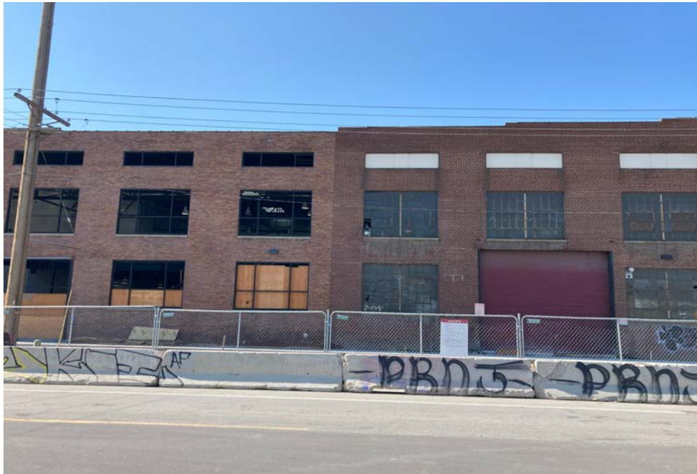
(Adjacent warehouse building used for inspiration for solid/void)
